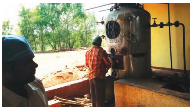
Plate 7.7: Mini boiler for steam generation
