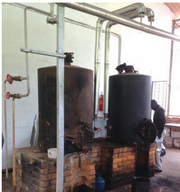
Plate 7.7: Mini boiler for steam generation
